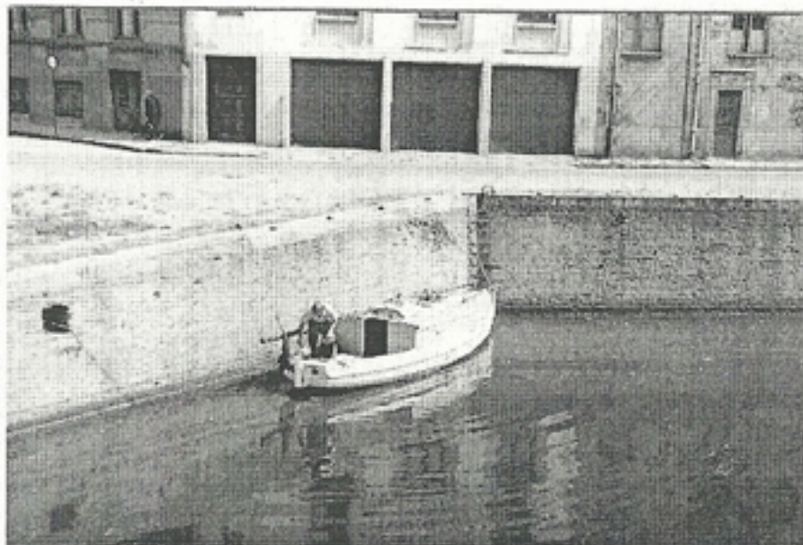
Re-fuelling in Dunkerque Mast un-shipped for canals
